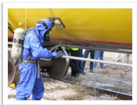
Responders patching the leak.
